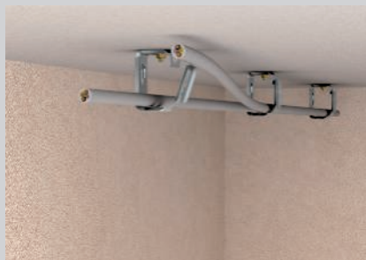
Opening of the grouped support and insertion of the cables.
