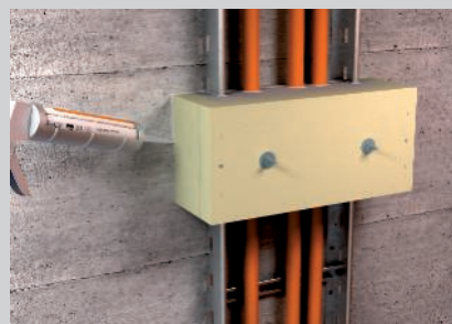
Closing all the remaining joints using the ASX fire protection compound.
