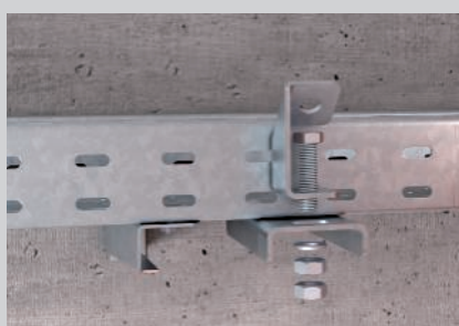
Fastening of the sloping connection component.
