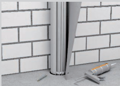
Installation of the fire protection bandage.
