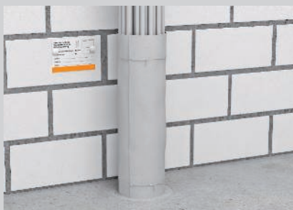
Using mortar, close off the residual insulation opening and mount the identification plate.
