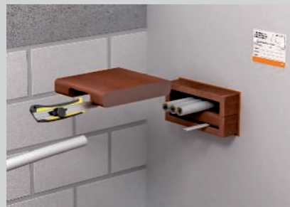
Exact cutting of the internal pieces and then insertion in the frame.
