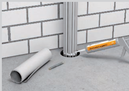
Preparation of the cable insulation.
