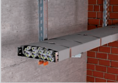
Complete encasement of the suspended cable run.
