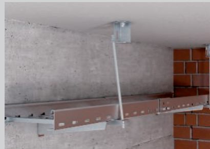
Ceiling fastening of the threaded rods with fire protection clamps.
