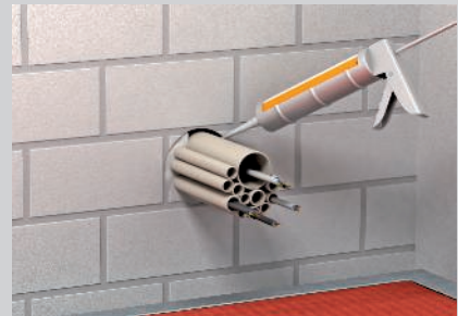
Closing of the ring gap with the insulation layer creator DSX.
