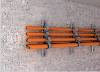
Horizontal cable mounting with clamp clips on the wall.
