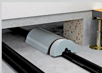
Adjusting the foam plug to the cables.
