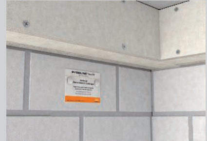
Labelling according to the VDE application rule.
