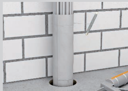
Fixing of the bandage using winding wire.
