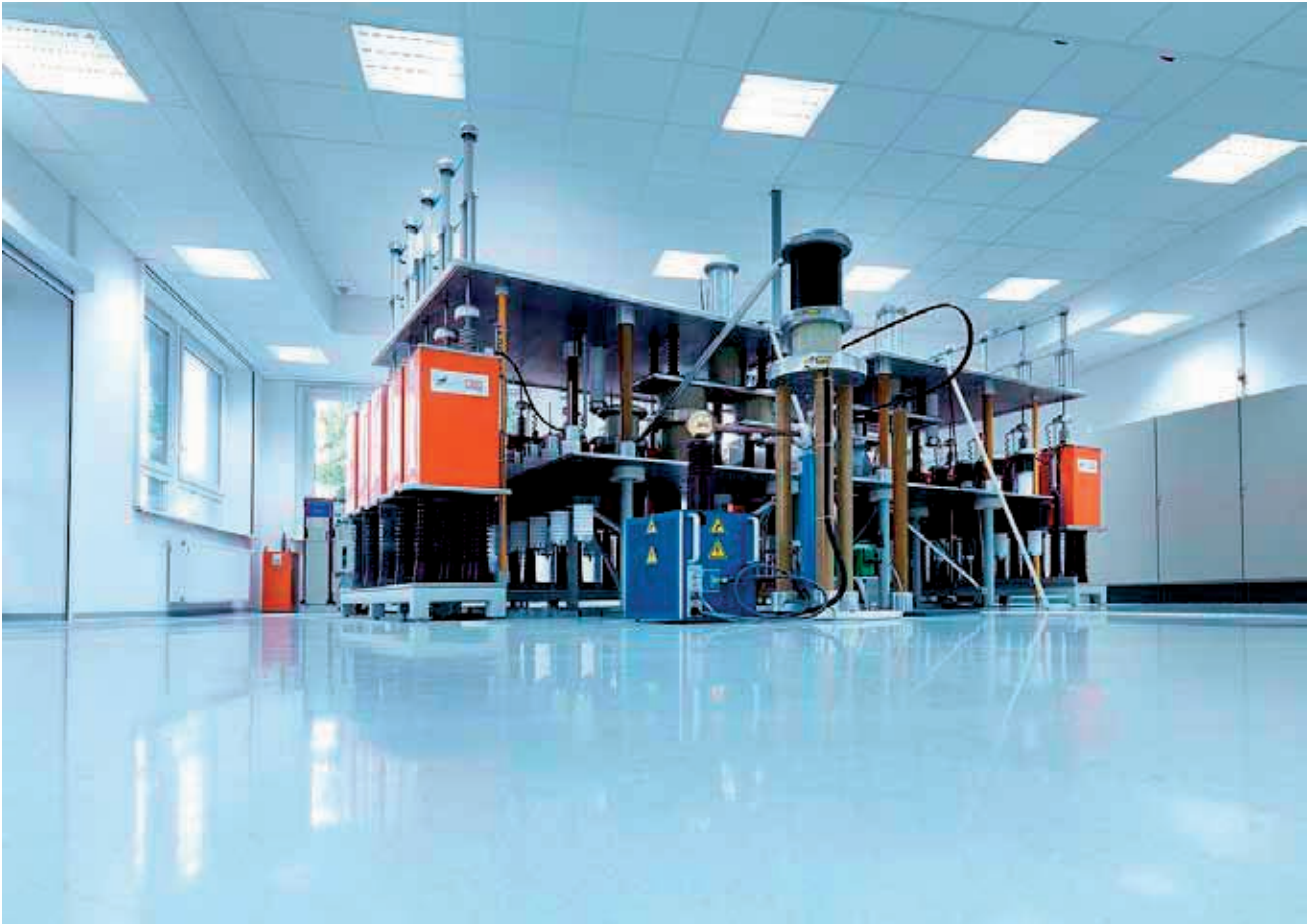
Lightning current generator
